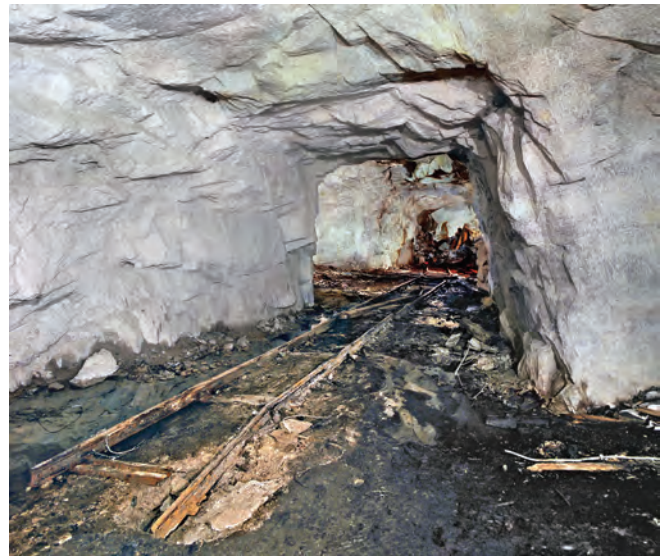
Rails are still in place in Ho 2 in a quarry at the base of Bluestone Hill overlooking The Nunnery. The tunnel was used for munitions storage.
